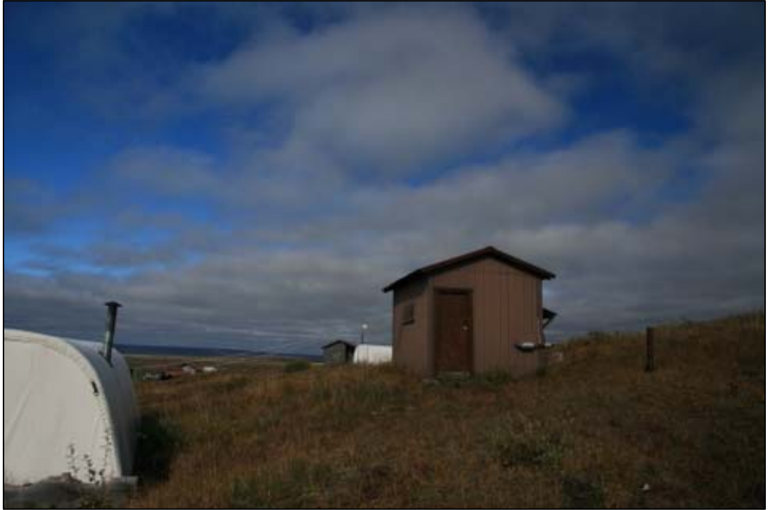
Photo 3 Generator shed from south.
