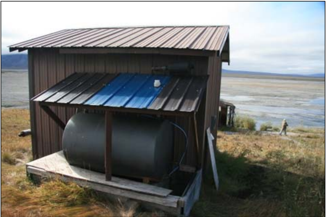
Photo 4 Generator shed from east.
