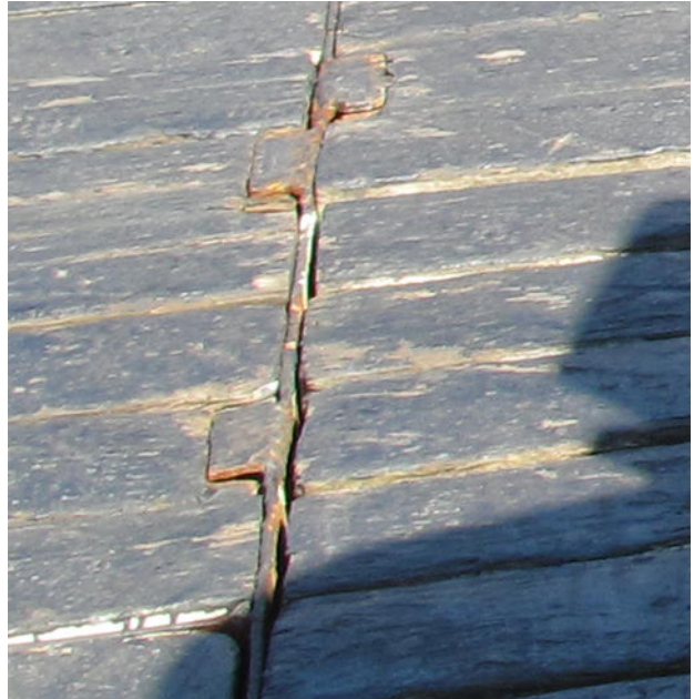
Figure 5-2: Typical Deck Hold Down Tabs
