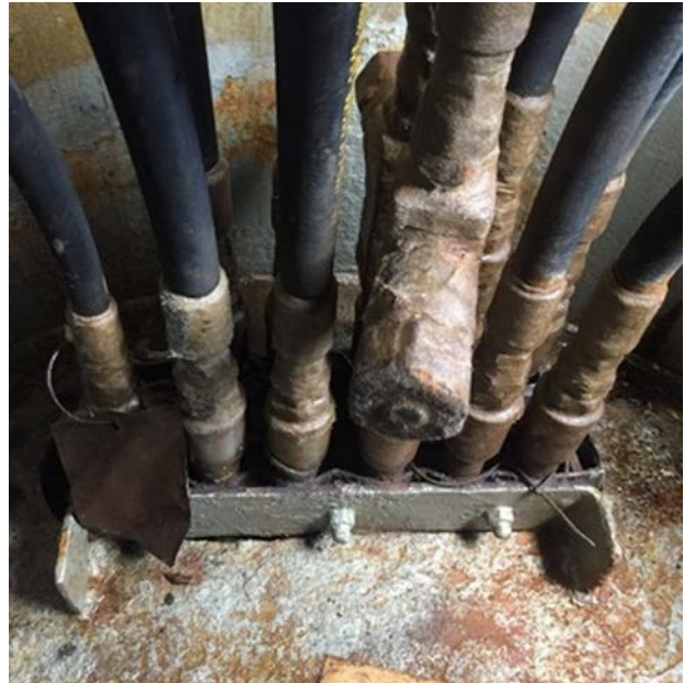
Figure 6-4: Hydraulic Hose Connections to Hydraulic Pipes Inside Pedestal Near Main Deck
