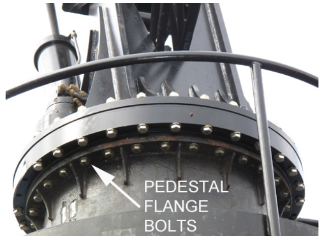
Figure 6-5: Existing Pedestal Flange Bolting
