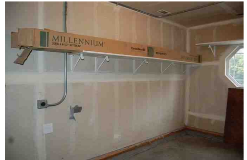
Garage Workshop Area
