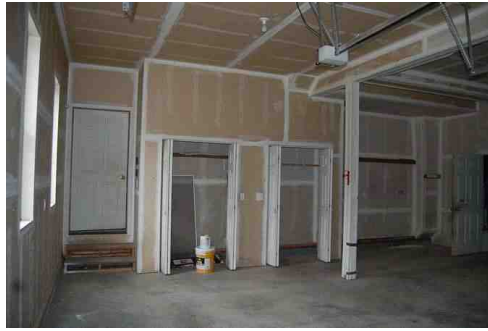
Garage Interior / Door to Entry
