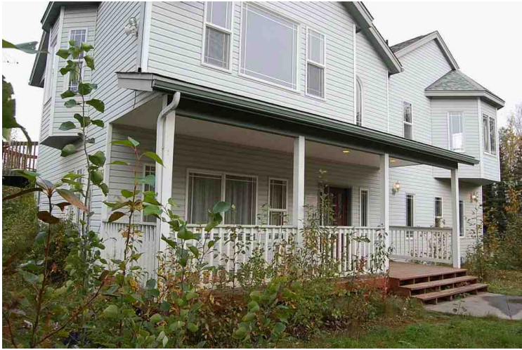
Additional Front Photo
