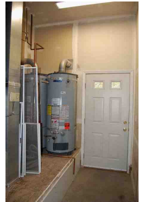
Rear Entry at Utility Room
