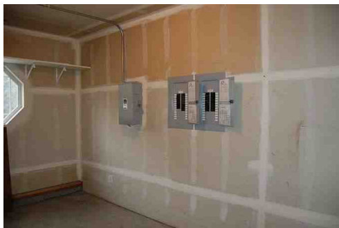
Garage Workshop Area
