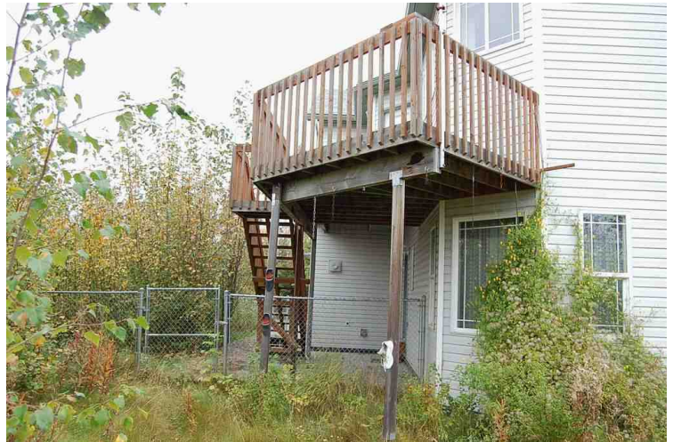
Northwest Corner Exterior Detail
