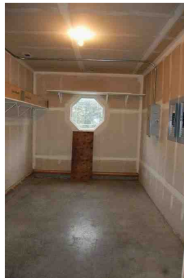
Garage Workshop Area
