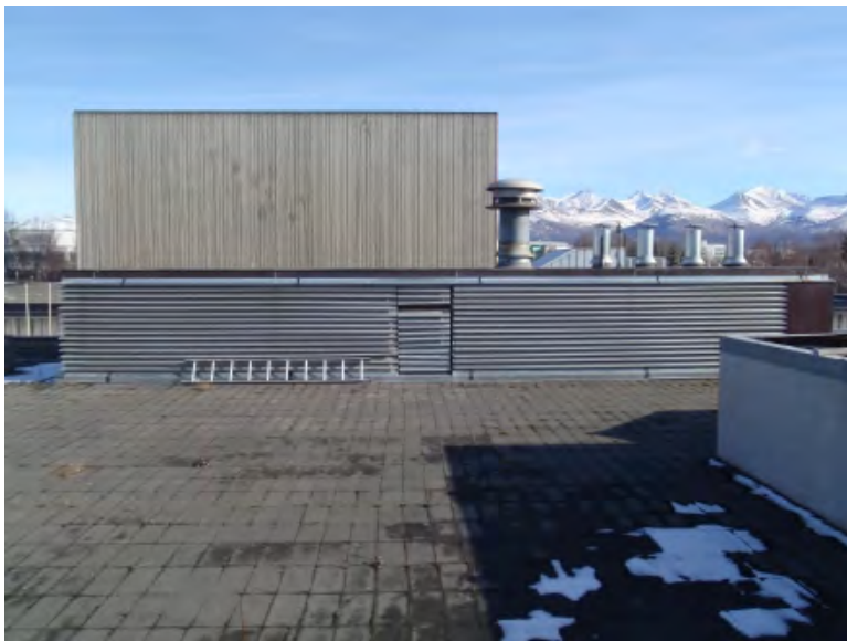
8. Facing east, penthouse with louvered walls.
