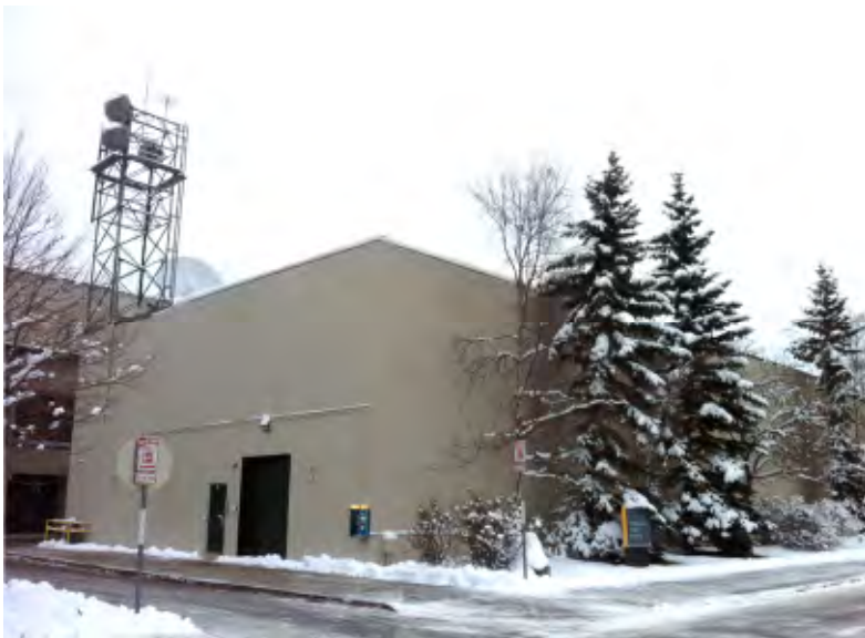
2. North & west sides of PSB at Roof 1.
