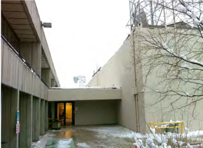
1. North entrance, Roof 3 center, Roof 1 on right.
