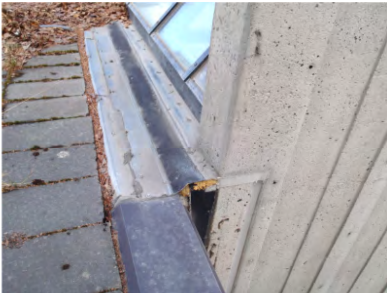
20. Roof 3, south end of building joint, facing north.
