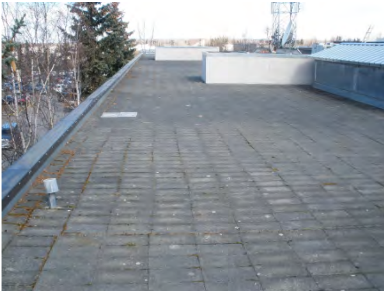
5. Facing north Roof 1.
