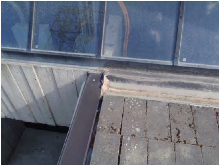
19. Northeast corner of Roof 3 with building joint.
