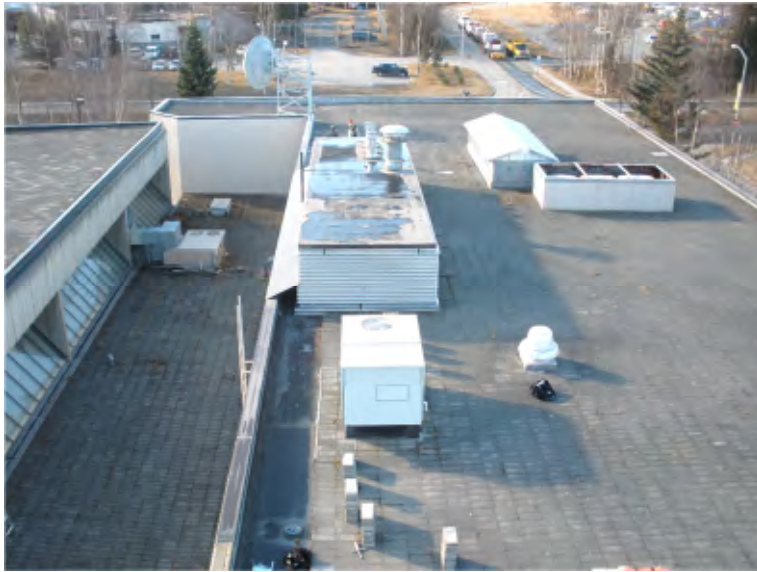
4. Facing south, Roof 1 on right.
