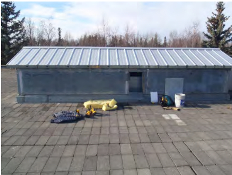
11. "Transfer duct" enclosure on Roof 1.
