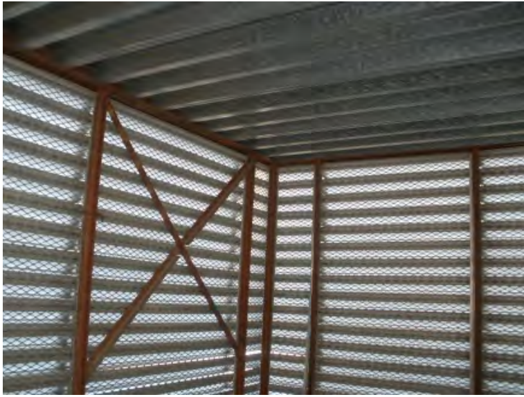
10. Penthouse interior louver wall framing, and underside of Roof 2 metal deck.
