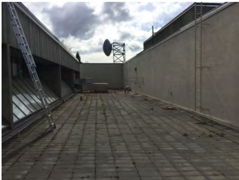
14. Roof 3, facing south. Note building joint at base of windows. (older photo).
