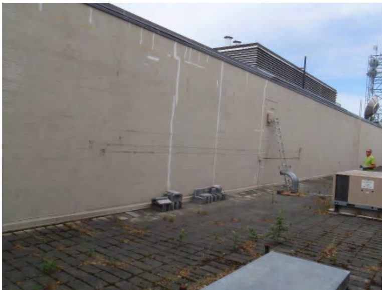
17. Roof 3, see photo 16.
