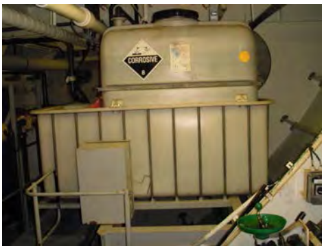
Figure 5- Chemical properly stored in a containment basin
