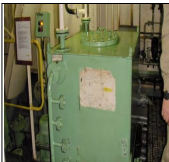
Figure 9: Example of pre-treatment system component "Sludge" concentration trunk tank
