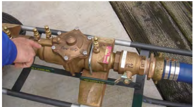
Figure 7: Backflow preventer
