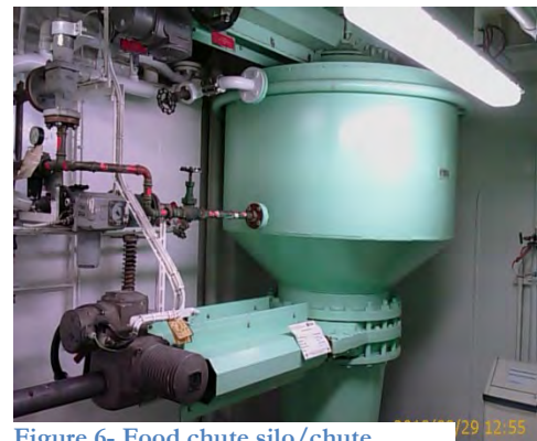
Figure 6- Food chute silo/chute
