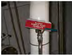
Example Zenon Permeate Sample Point (close-up)
