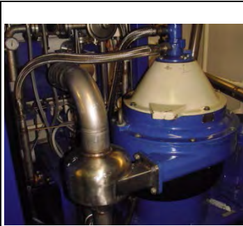
Figure 11: OWS separator / sludge treatment (dynamic) "concentrator"
