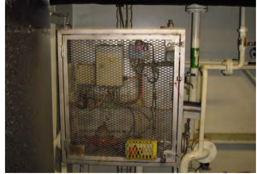
Figure 8: Example Large Vessel OWS / White Box System
