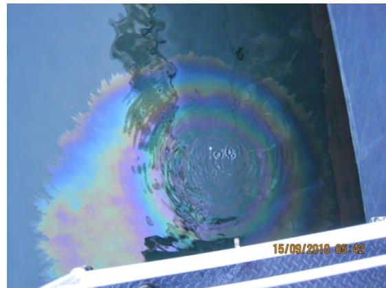
Figure 2- Small spill from ruptured hydraulic line
