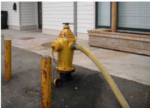
Figure 4 Example potable water source
