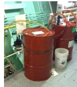
Figures 21 and 22: Temporary Oil filtration or pumping system
