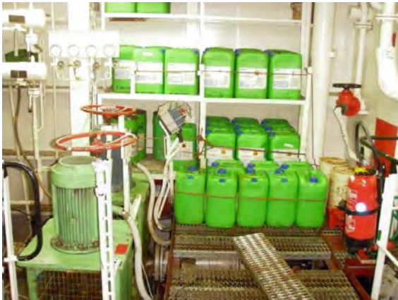
Figure 5- Chemical properly stored in a containment basin
