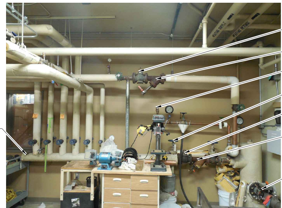
DOMESTIC WATER SUPPLY HEADER
