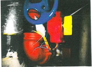
YES NO NA ALARM-RECEIVING FACILITY RECEIVES SIGNALS PROPERLY? THERE WERE 109 TROUBLE SIGNALS PRESENT ON THE PANEL UPON ARRIVAL. NO ALARMS SIGNALS WERE RECEIVED BY THE ALARM RECEIVING FACILITY EVEN THOUGH ALARMS SHOWED UP ON THE ALARM PANEL. THE PENTHOUSE & 7<sup>TH</sup> FLOOR FLOW SWITCHES DID NOT SEND ALARM SIGNALS TO THE ALARM PANEL WHEN WATERFLOW OCCURED.
