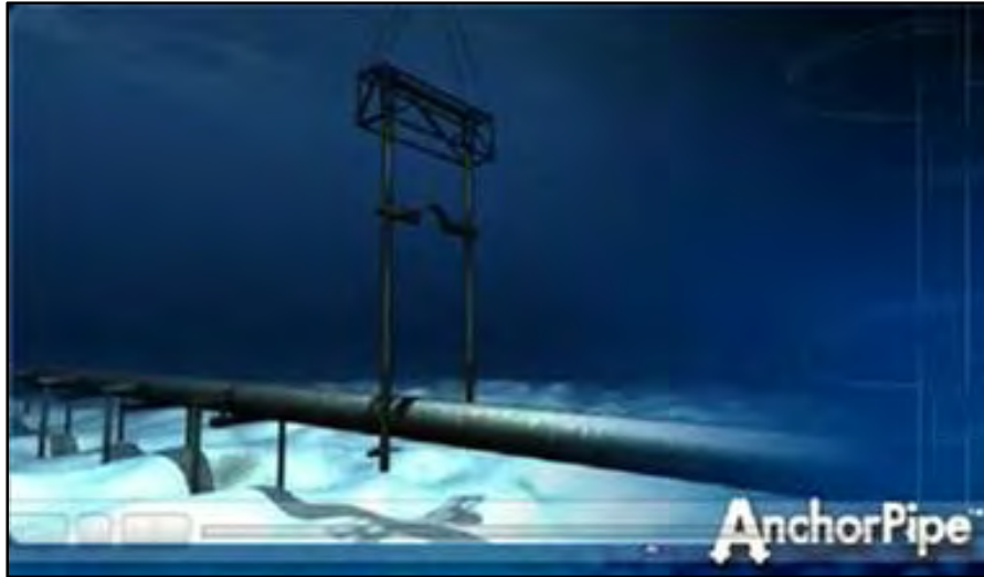
Photo 4: Anchor Installation Example
