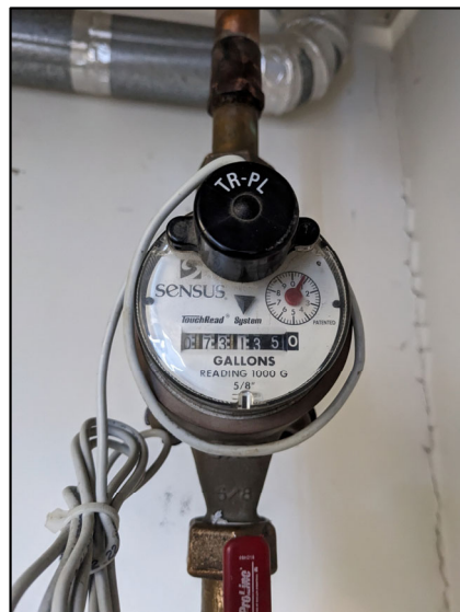
Water meter post pressure tanks going to distribution.
