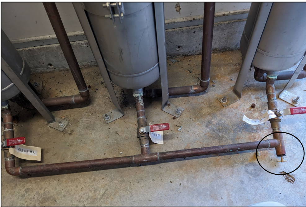
Filter drain capped following 2018 sanitary survey.
