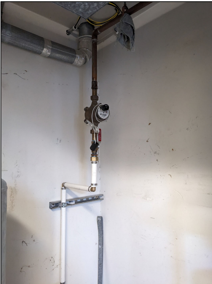
Water meter post pressure tanks going to distribution.
