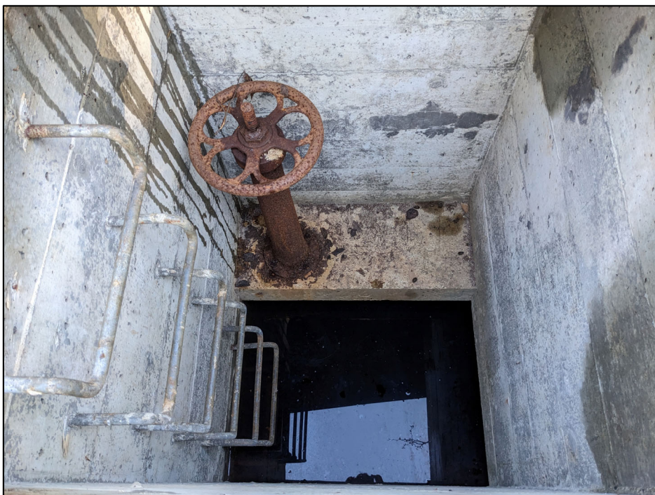
Inside of vault #2, water was 7 ½ feet deep, vault is 14 feet deep.
