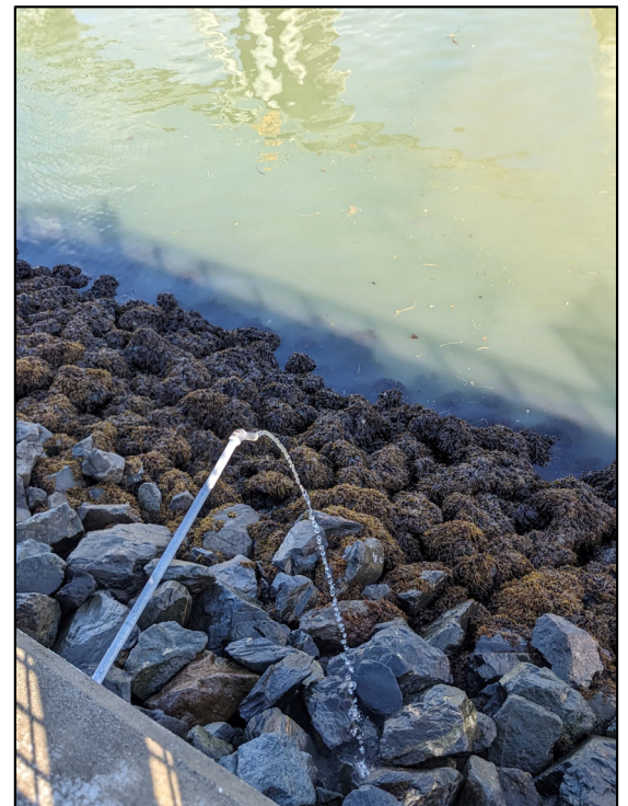
Pipe runs to breakwater wall and discharges. Discharge point is located above high tide line.
