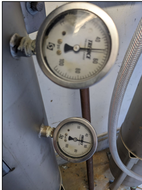
Pressure gauges for filters 1, 2, and 3.
