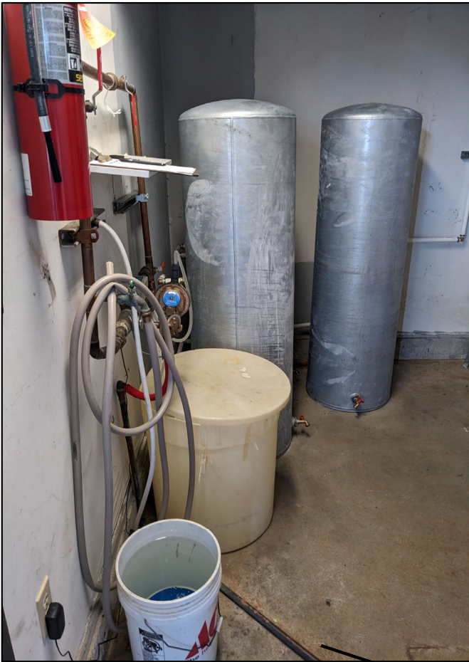
All 3 tanks were replaced in August 2023 with Quick Tanks, Inc. Q82V 82-gallon galvanized vertical tanks with NSF standard 61 lining.
