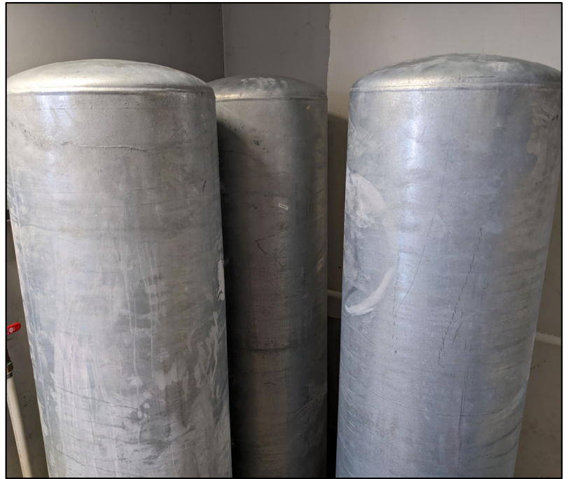
All 3 tanks were replaced in August 2023 with Quick Tanks, Inc. Q82V 82-gallon galvanized vertical tanks with NSF standard 61 lining.
