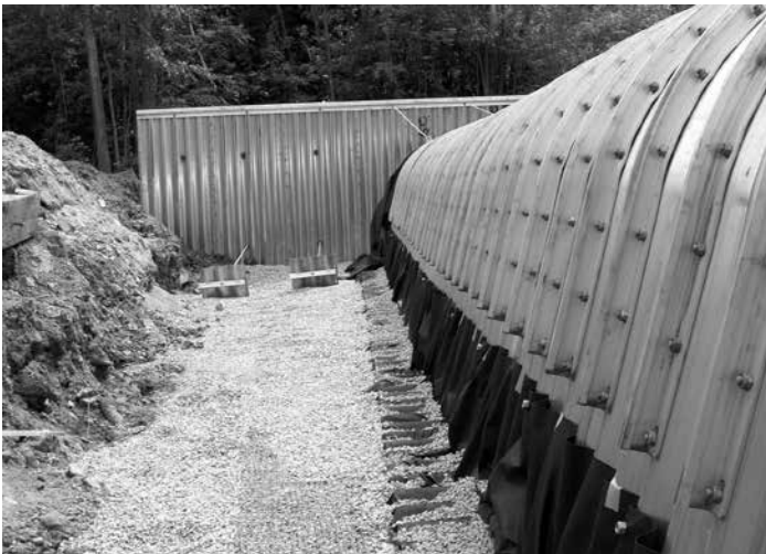
Loosely placed geotextile over scallop plate and exterior of invert plate.
