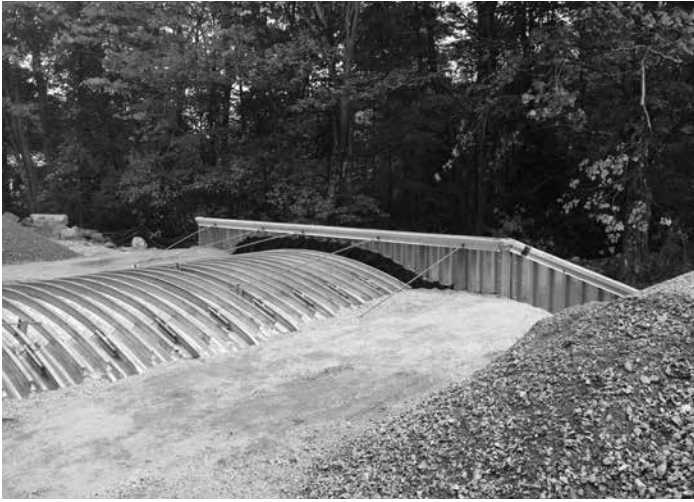
Granular material placed in balanced manner.
