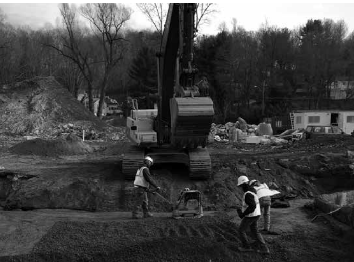
Backfill material is placed and spread from a distance with an excavator, then compacted with a vibratory plate compactor.
