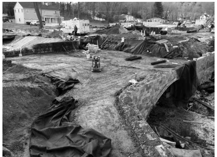
Backfill material is placed and spread from a distance with an excavator, then compacted with a vibratory plate compactor.
