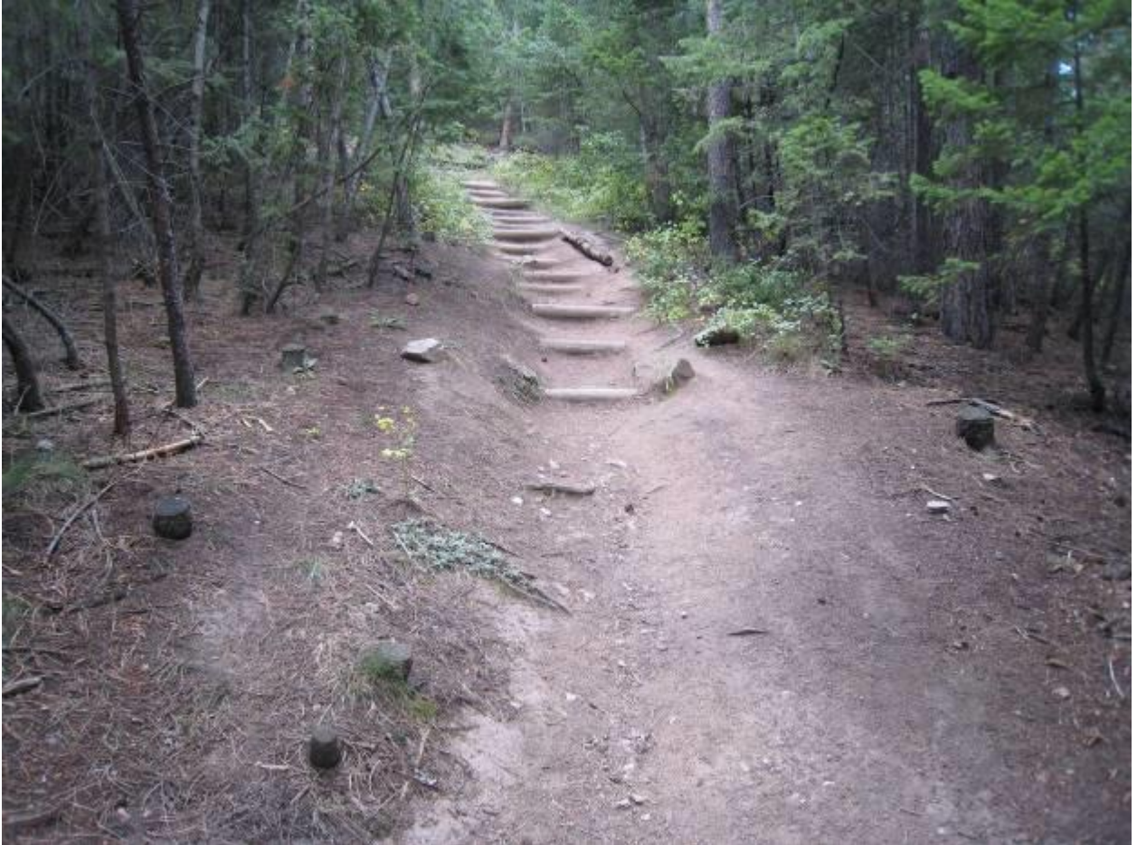
Example of step construction using pressure treated turned logs. This is on Green Mountain in Boulder Mountain Parks in Colorado.
